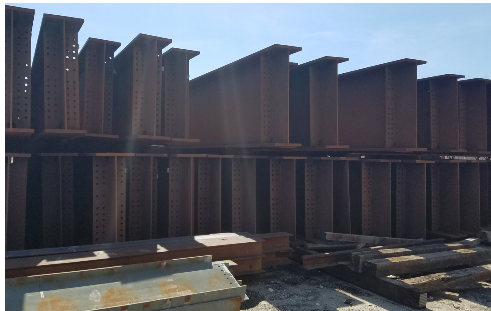
Figure A5.2.8-7: GLP will reuse 100% of the MBTA-provided materials including steel located at Casco Bay for the construction of the Lechemere Viaduct.
