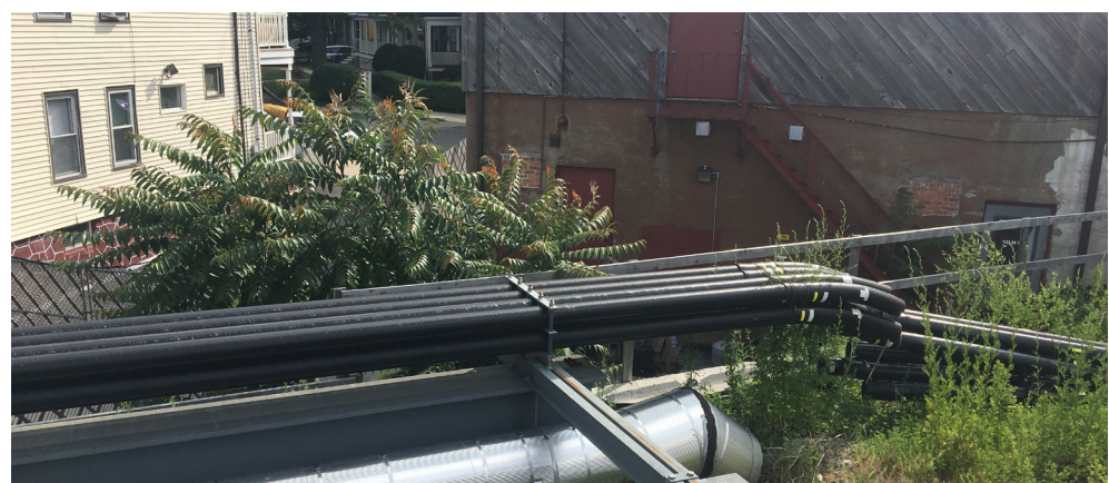
Figure A5.2.9-5: Transitions of water, power and communications lines from underground to the utility bridge. GLP will convert the temporary utility bridge to permanent, thereby reducing the cost and service interruptions to customers associated with relocating utilities back to the roadway bridge
