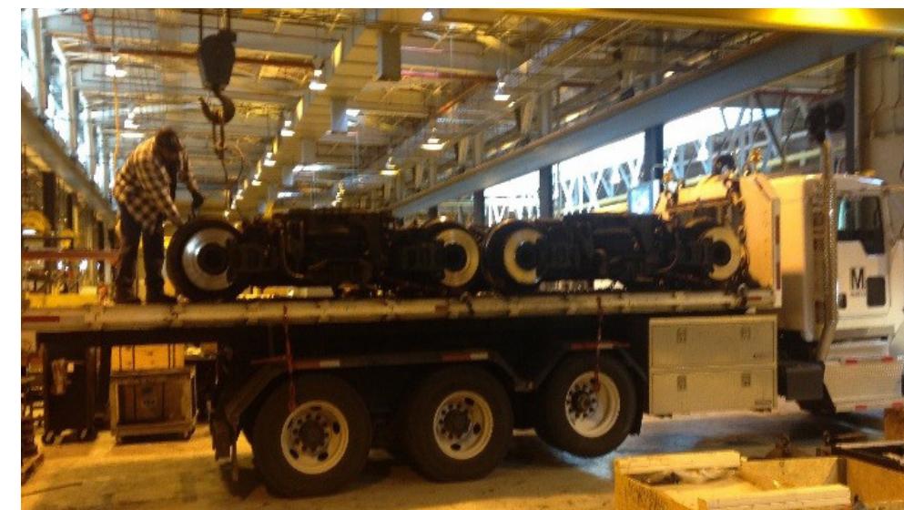
Figure A5.2-7: GLP has designed a loading bay configured to allow a bridge crane to load and unload a powered truck, the heaviest LRV component, from a flatbed truck. This efficient design will accommodate the material handling of all LRV components.
