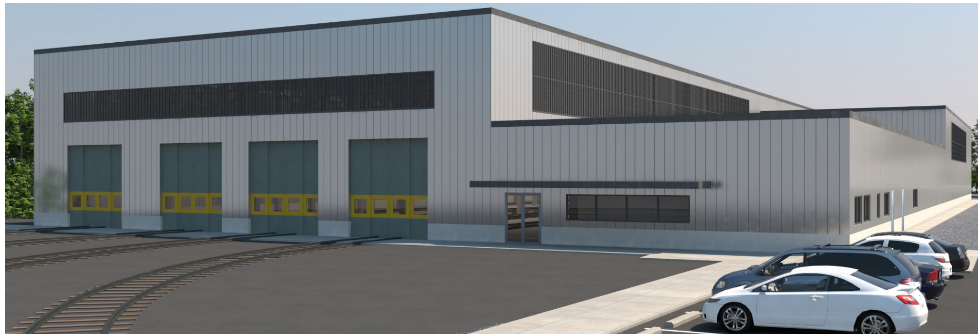
Figure A5.2.5-1: GLP's proposed VMF building design allows for more efficient and safe operations by relocating welfare spaces close to the parking, eliminating the need for staff to walk through yard operations.
