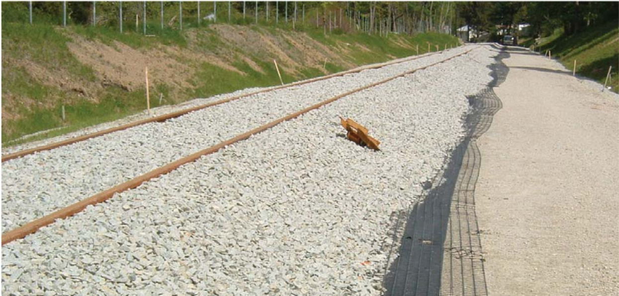
Figure ATC-43-2: MBTA Greenbush Line Construction
