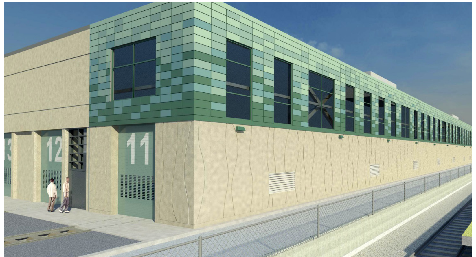
This is similar to the Wellington Carhouse Project that GLX Constructors' Lead Designer, STV, recently completed design on. The Carhouse, another utilitarian building, is immediately adjacent to the Wellington subway platform. The use of colorful metal panels and textured precast concrete panels gives a nod to the local river in their design, and presents an interesting face to the users of the station.
