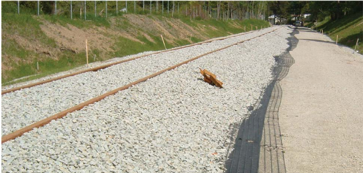
Figure ATC-43-2: MBTA Greenbush Line Construction
