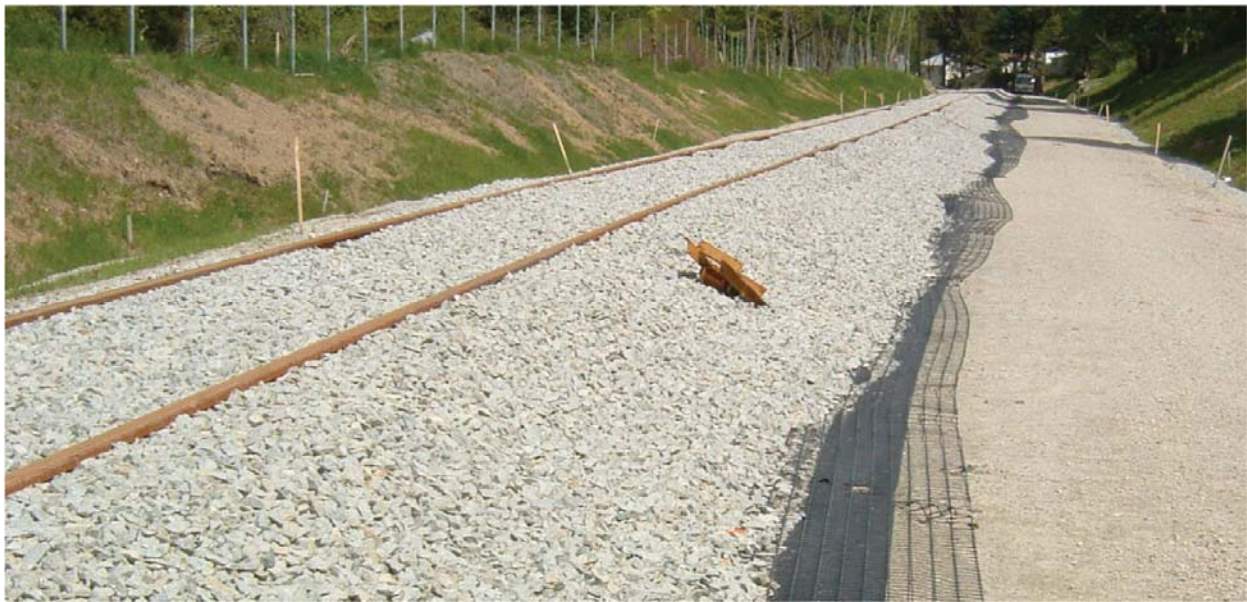
Figure ATC-43-2: MBTA Greenbush Line Construction
