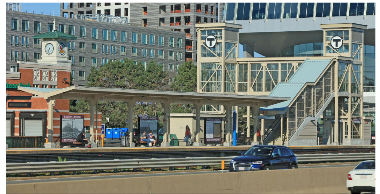
Figure 1-1. MBTA Boston Landing Commuter Rail Line Canopy. The wing-style canopy used will be adapted for this Project to extend the wings of the canopy 5-1/4 feet beyond the edge of the platforms.
