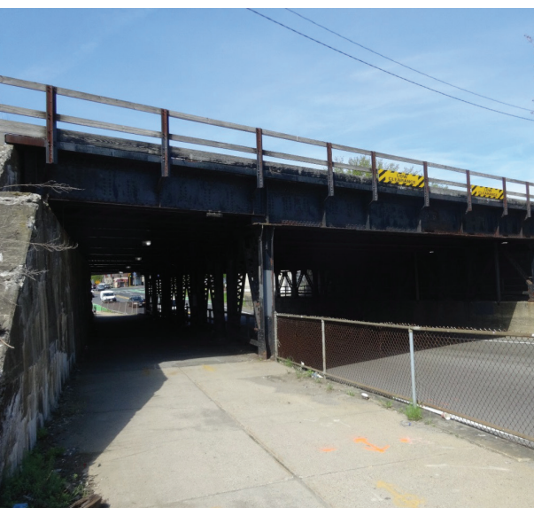
Figure 4.2-17. Washington Street Bridge. Our approach is to replace the existing three-span bridge with a new single span superstructure which will provide better lighting and access for pedestrians.
