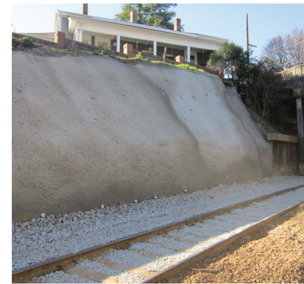
Figure 4.2-9. Permanent Soil Nail Wall. Soil nails provide an efficient structural solution where ROW is available.
