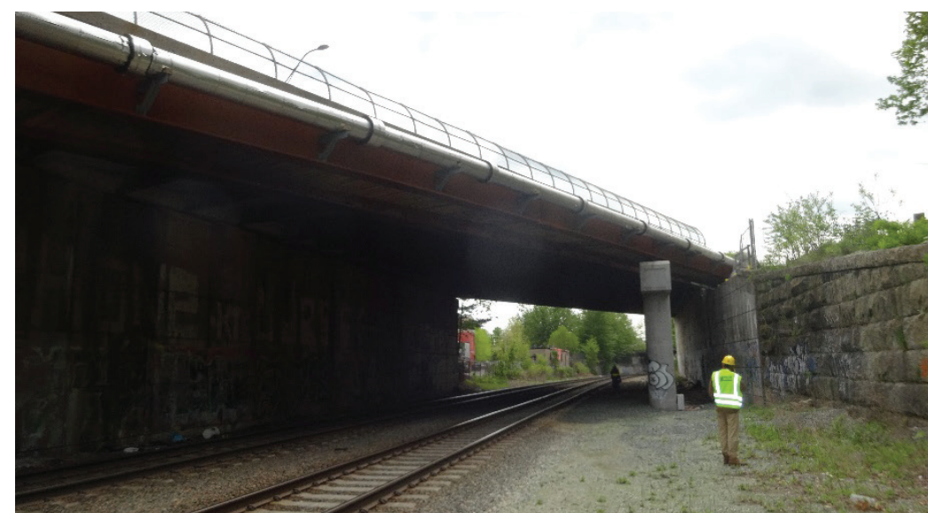
Figure 4.2-18. Medford Street Bridge. Our approach to modifying the existing bridge retains the existing superstructure, modifies the bridge seat, and the constructs a new back span.
