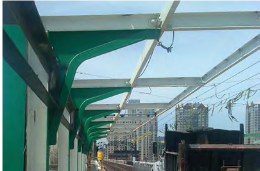
Existing Sign Frames
