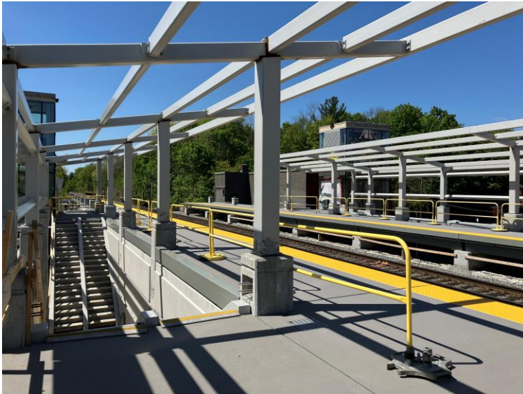
Platform and stairway at the Aberjona side of the Headhouse
