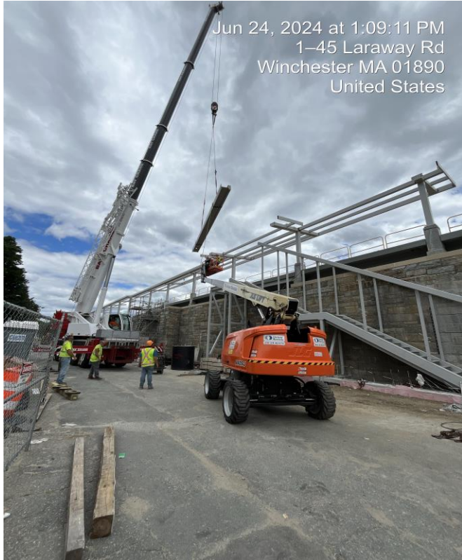
Laraway Road stair installation
