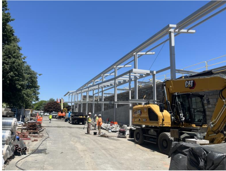
View of the Station along Laraway Road
