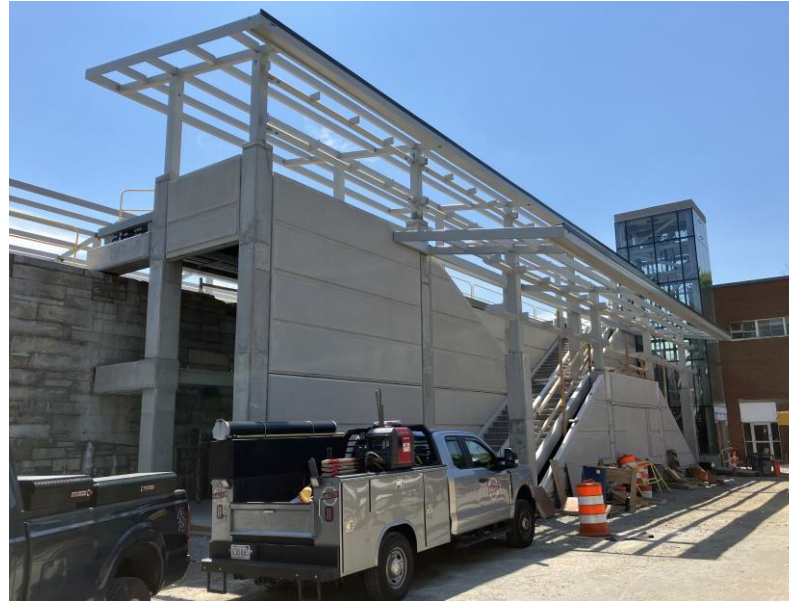
Waterfield Lot side of the Headhouse
