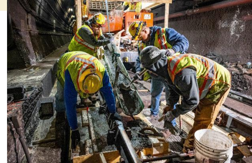
Repairing concrete slabs
