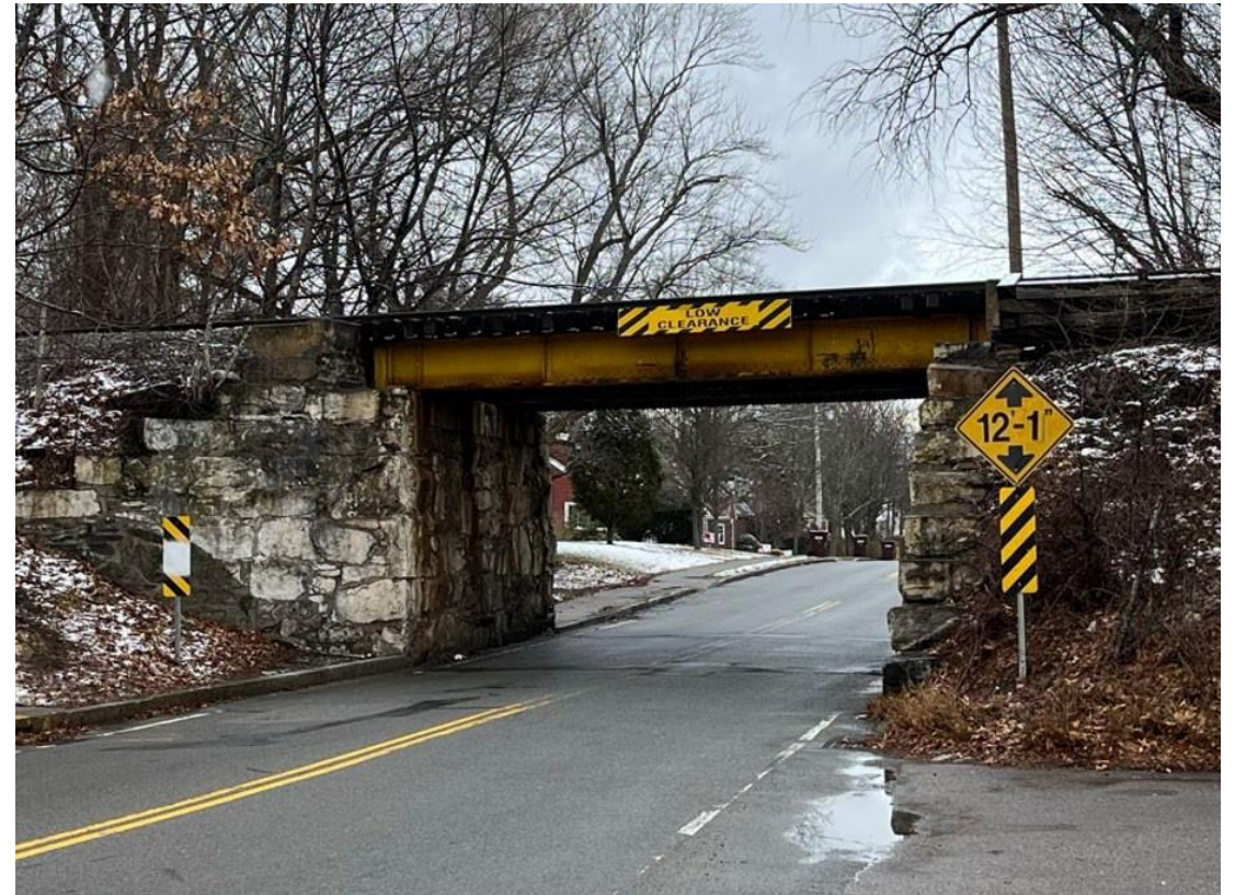
East St. Bridge – West Elevation
