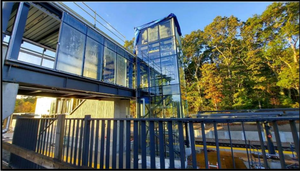
East Taunton Station under construction
