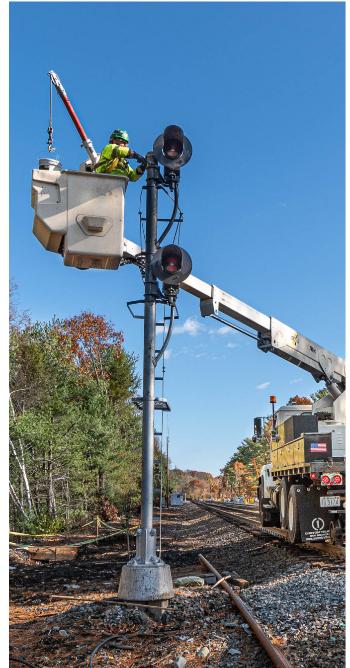
Crew member installing new Commuter Rail wayside signal equipment in Weston..
