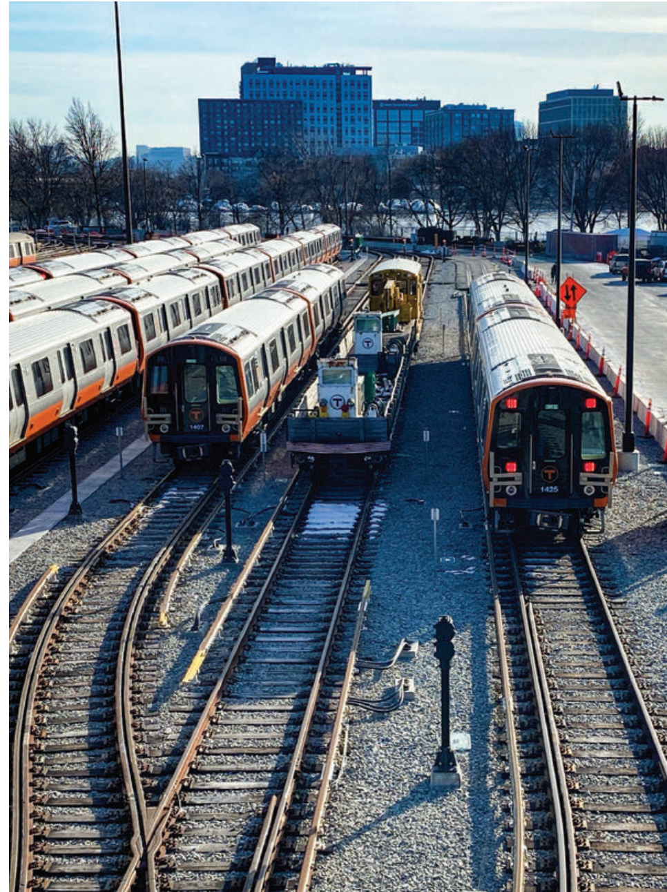
New Orange Line heavy rail cars and maintenance equipment at Wellington Yard.
