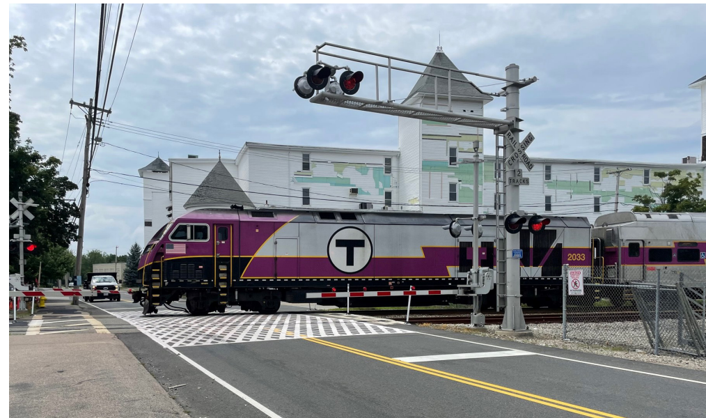
Grade crossing at Plymouth Street on the Kingston Line in Abington.
