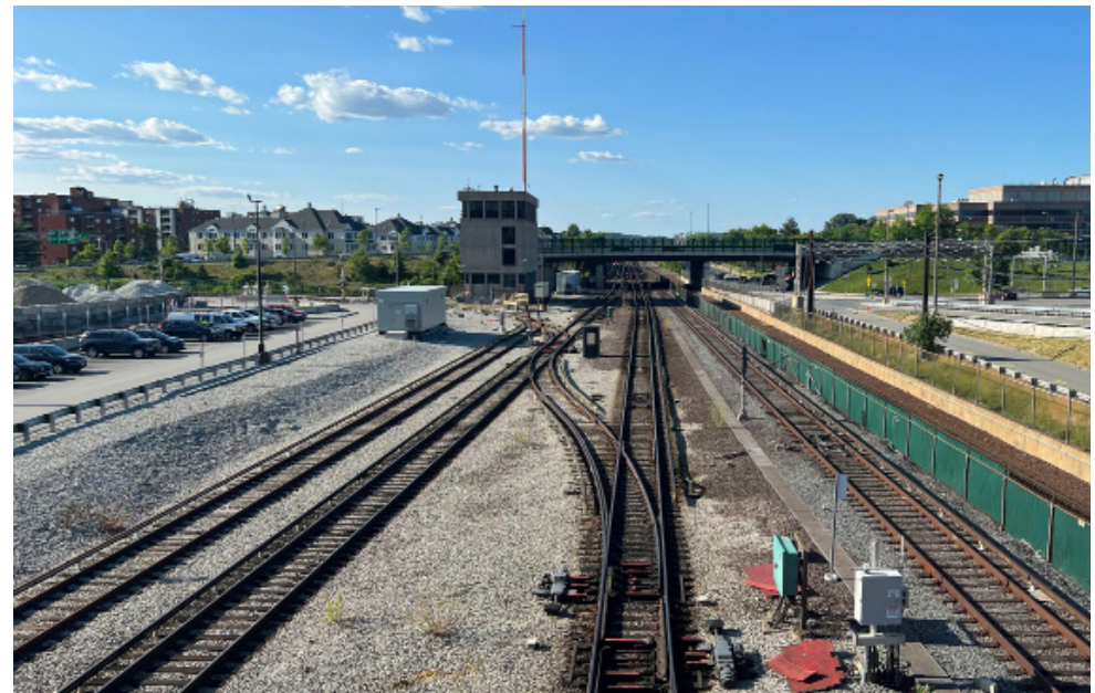
Orange Line track turnout near Wellington Station.
