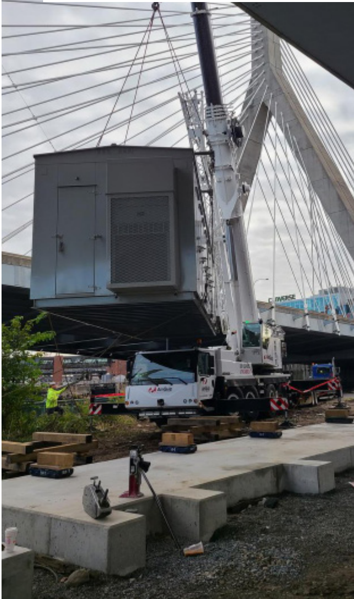
A signal house being installed near North Station.
