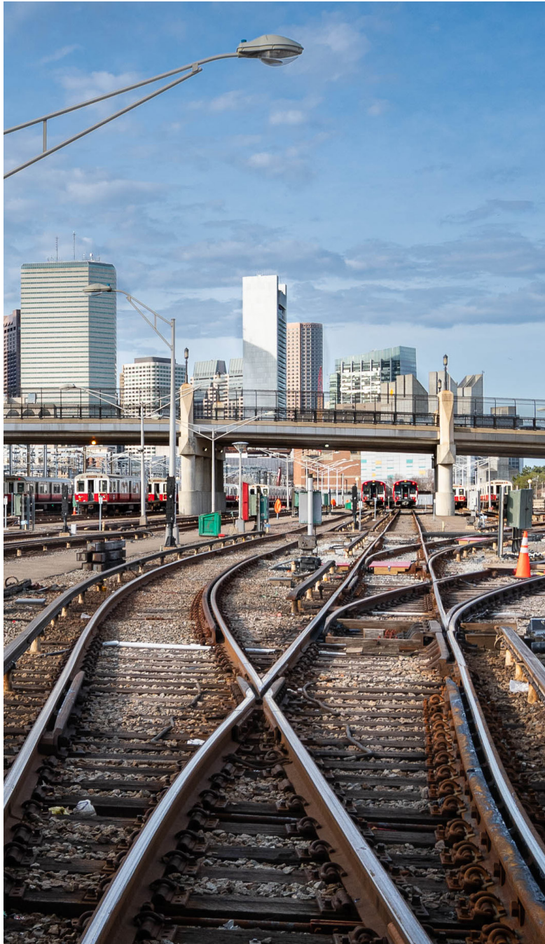
Interlocking at Cabot Yard on the Red Line.
