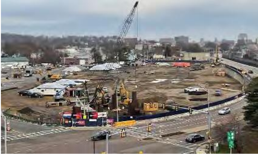
New Quincy Bus Maintenance Facility
