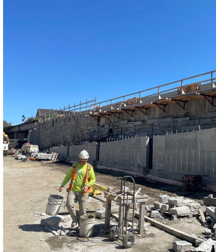
Inbound Ramp Construction – Laraway Road (September 2023)
