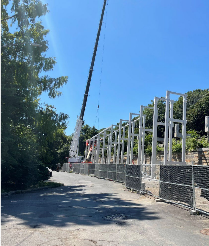
Ramp AA Structural Steel – Aberjona Parking Lot (September 2023)
