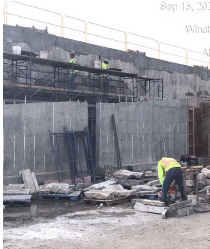
Wall Construction along Laraway Road (September 2023)
