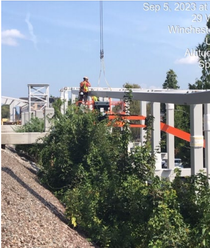
Outbound Platform – Steel and Concrete Construction (September 2023)
