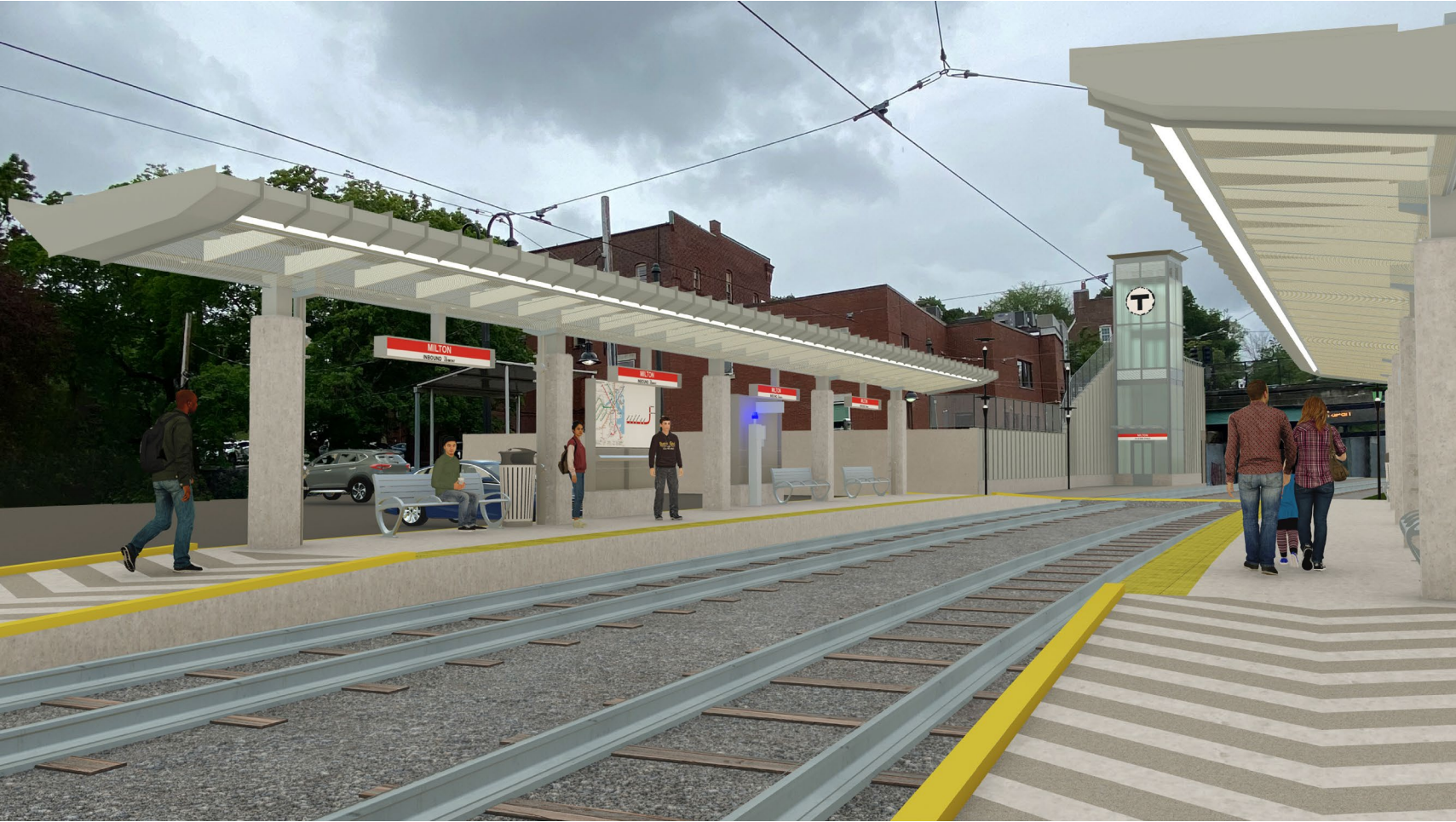
Proposed platform configuration at Milton Station with an elevator from the inbound platform to Adams Street
