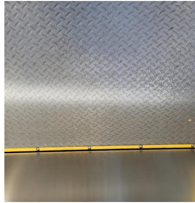
Non-Skid Surface in Vestibule
