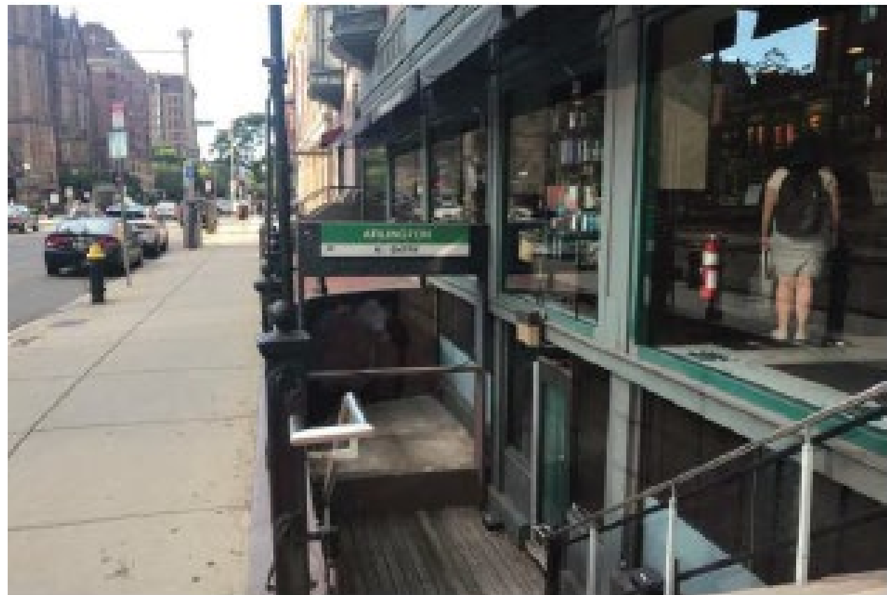
Exit only stairs at Berkeley street currently closed
