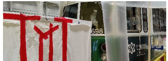
Abatement ongoing on 3600 series vehicles
