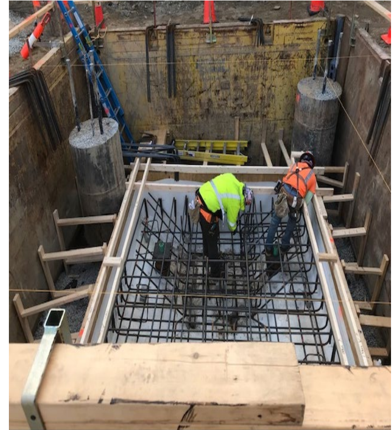
Elevator Foundation at Aberjona Lot (October 2022)
