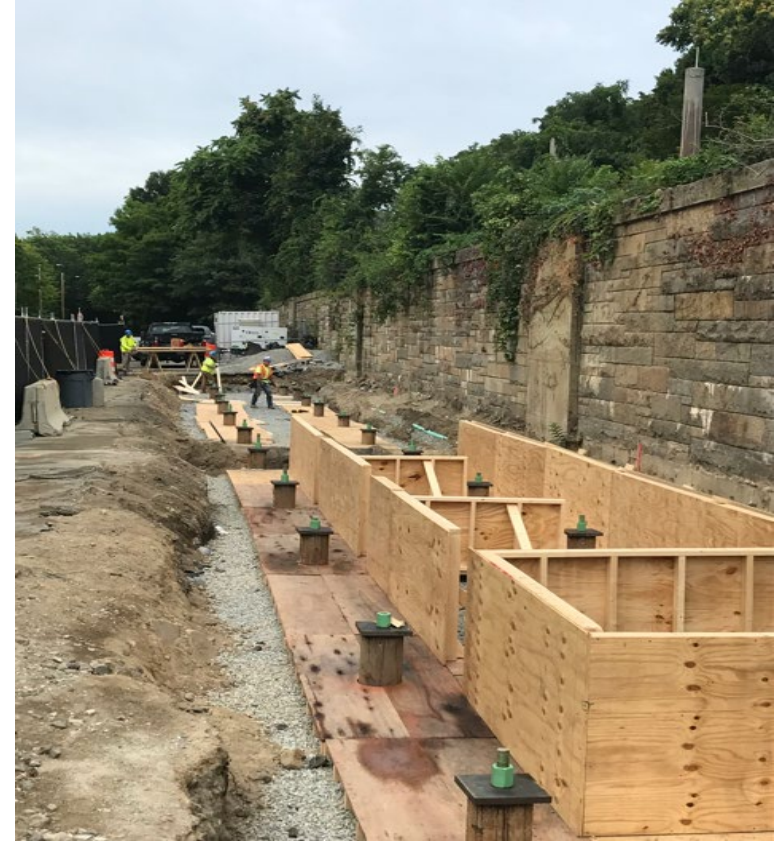
Forming Pile Caps and Grade Beams at Aberjona Lot (August 2022)
