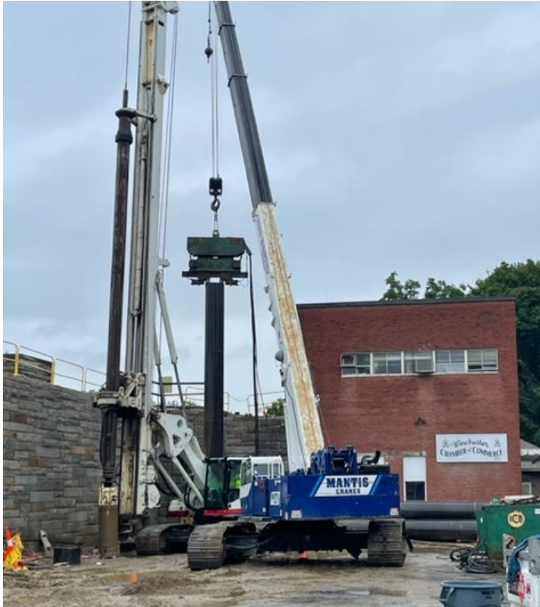
Drilled Shafts for Elevator at the Waterfield Lot (September 2022)
