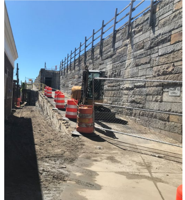
Demolition at Northeast Ramp behind the Thompson Street buildings (September 2022)
