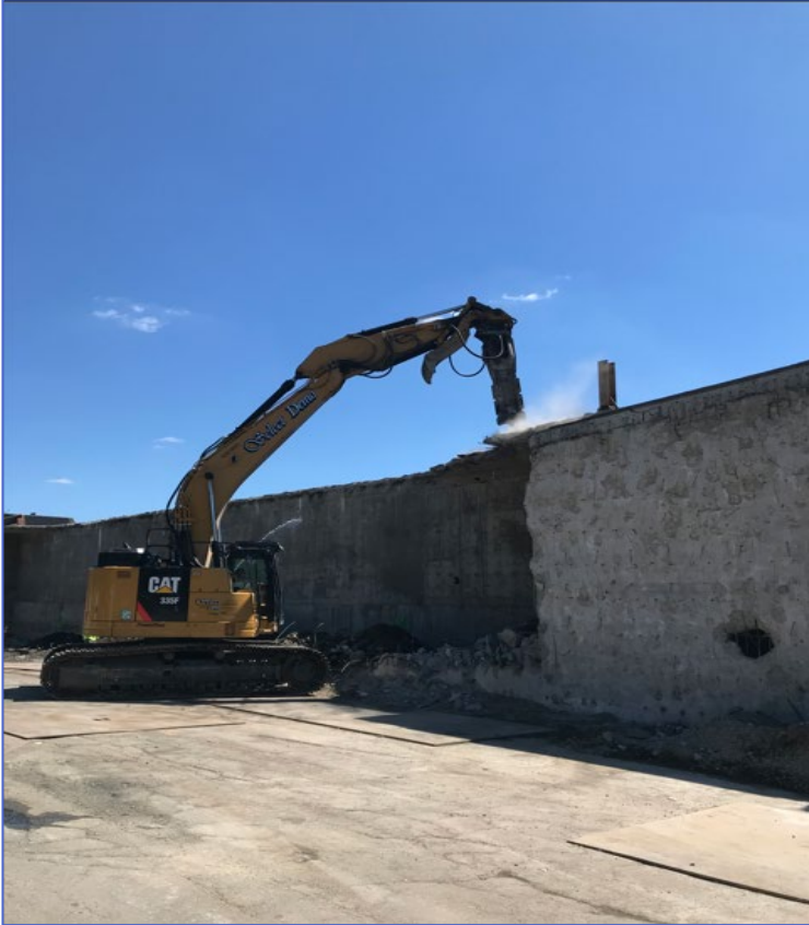
Demolition Work at the Laraway Lot (July 2022)
