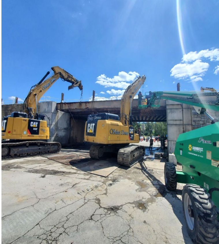
Demolition Work at the Waterfield Bridge (July 2022)
