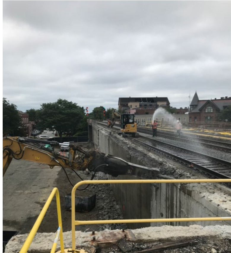
Granite Stone Removed and Demo at Laraway Lot with dust control (August 2022)
