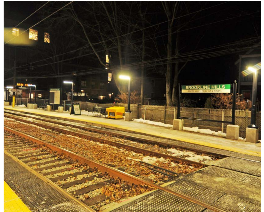
New Lighting Platforms, Walkways & Parking
