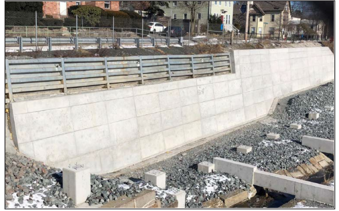
Completed retaining wall shown above, completed in December 2021.
