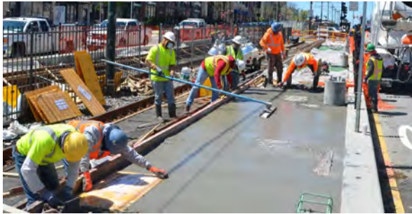
B Branch Consolidation two new accessible stations
