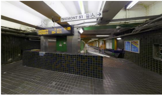
Park Street existing conditions
