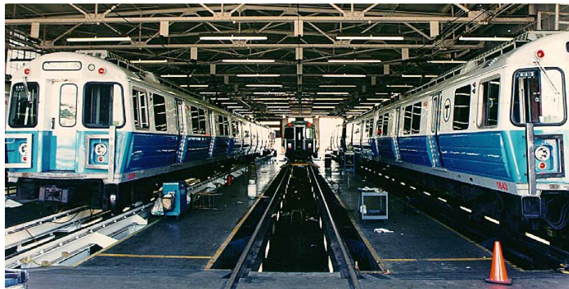
Orient Heights Maintenance Facility (Blue Line Service)
