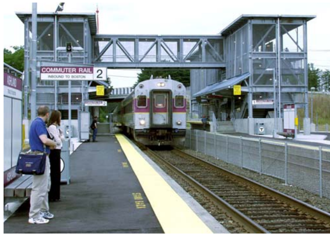
Ashland Station (Worcester Line).
