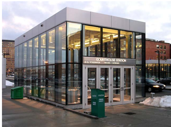
Courthouse Station (Silver Line)
