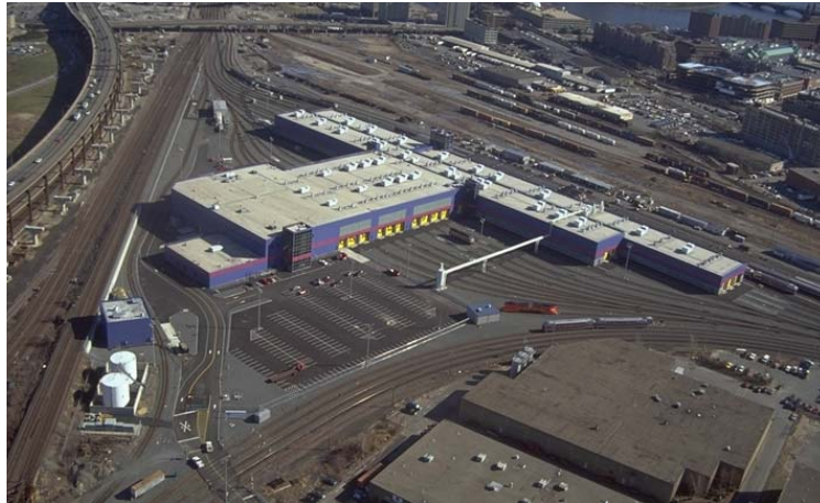
Boston Engine Terminal
