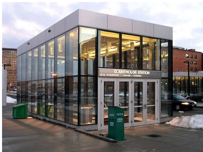
Courthouse Station (Silver Line)
