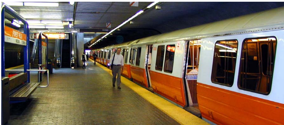
Forest Hills Station (Orange Line)
