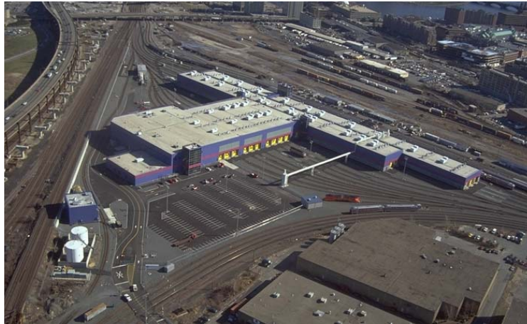
Boston Engine Terminal
