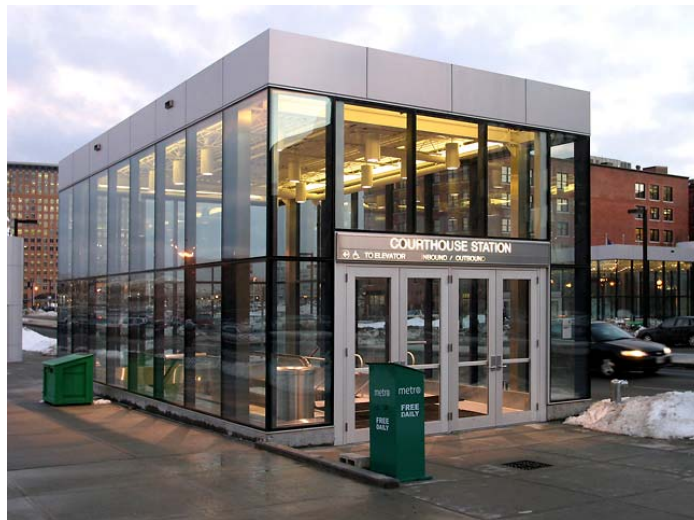
Courthouse Station (Silver Line)
